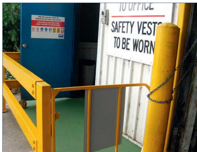
AFTER: Solid barrier with gate installed.
